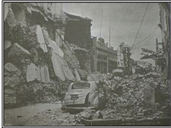
View of the earthquake damage San Juan which destroyed the city
